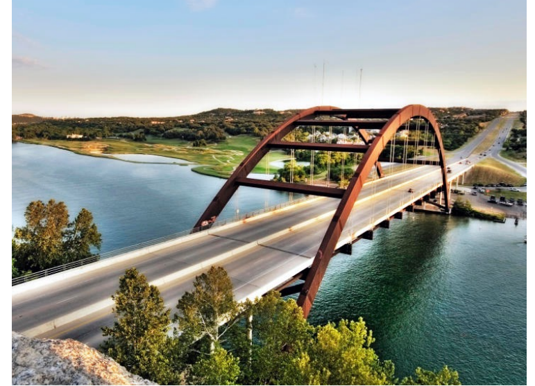
Pennybacker Jr. Bridge in Austin, Texas (Rusty Colour)
